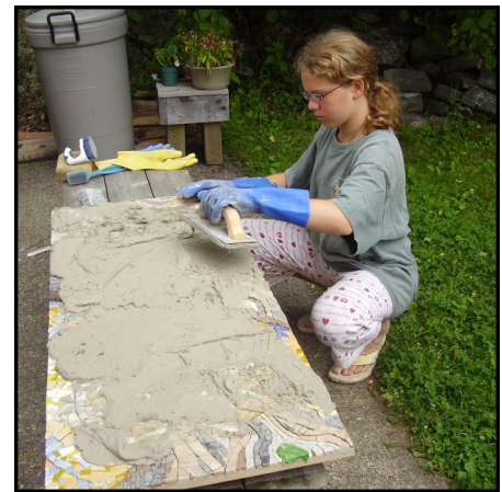
Using a grout float to force grout between the tiles. Messy!!
